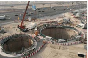
Deep Tunnel Storm Water System Dubai
