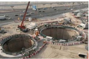
Deep Tunnel Storm Water System Dubai
