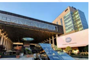
Extension of the Iulius Shopping Center Timisoara
