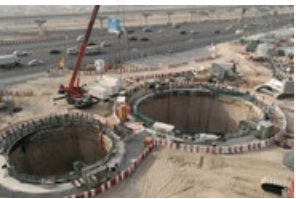
Deep Tunnel Storm Water System Dubai
