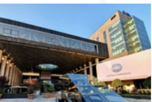
Extension of the Iulius Shopping Center Timisoara
