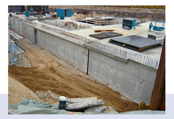
With the RASCOtank Complete Waterproofing Concept, the structural concrete doubles up as waterproof barrier.
